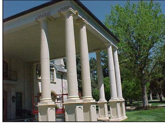
3 pillars on left- completed
