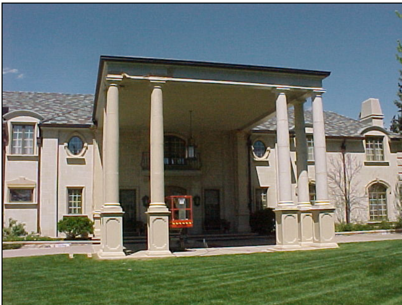
After 2 pillars on left completed
